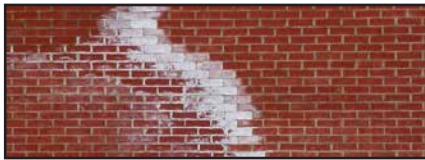
Cleaning & Descaling Before After
