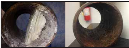
Drains Before After
